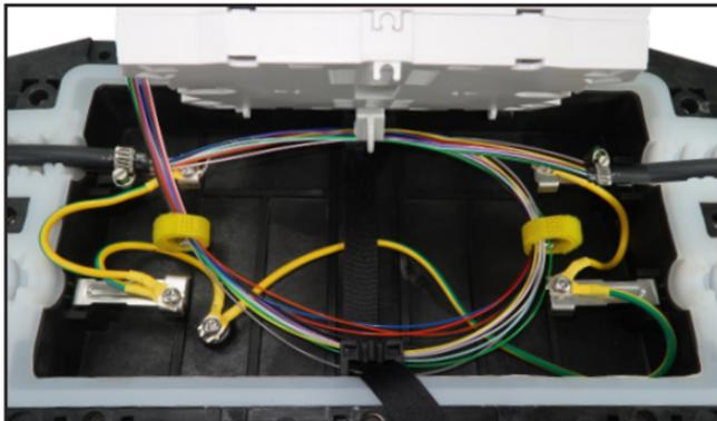
Figure 1-11: Install pass-through cable through other cable entry
