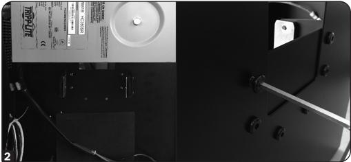
Reinstall and secure the U-shaped bracket to the outside of the enclosure using the hex key and the screws from the previous step. Secure the screws from the inside of the enclosure.
